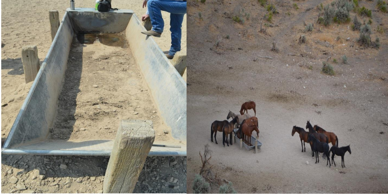
Figure 29. Cherry spring trough in August 2016 left and August 2017 on the right. Wild horses had damaged the support beams on the trough. No measurable flow of water. The spring was producing <1 gallon/hour.
