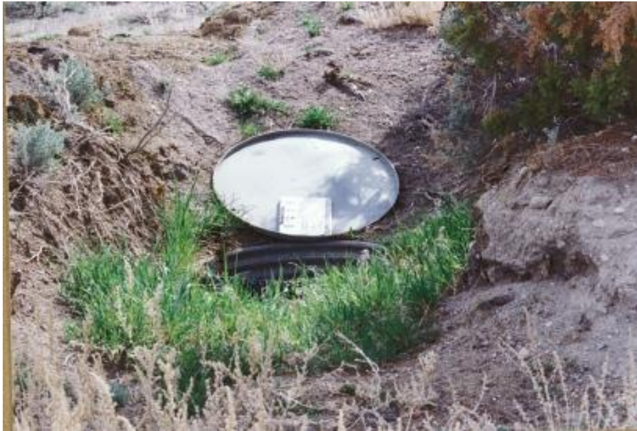
Figure 25. Sheep Camp spring, Goshute Mountains, spring development diverting most of available flow to a trough for wildlife and wild horses. Livestock season of use is from 11/1 to 4/30.
