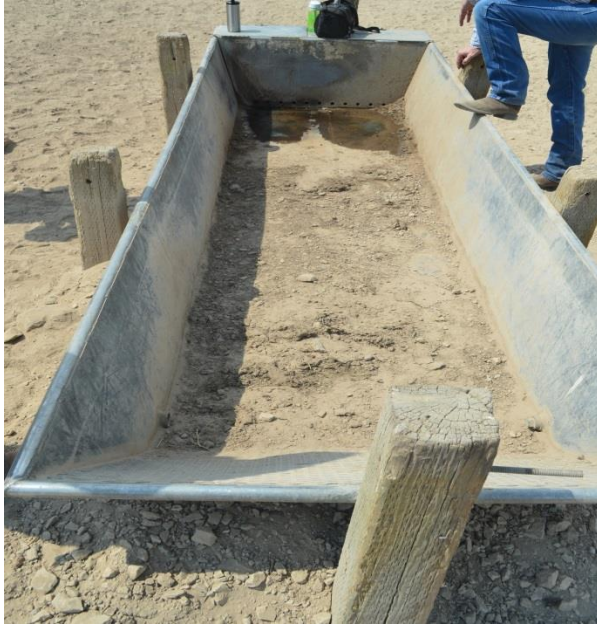
Figure 4. Cherry spring trough in August 2016. Wild horses had damaged the support beams on the trough. No measurable flow of water. The spring was producing <1 gallon/hour.
