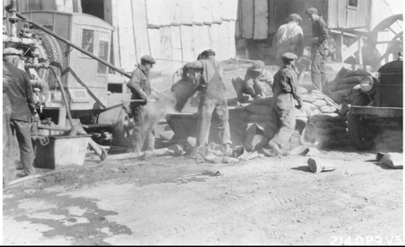
Perkins Cementing Outfit, running 750 sacks of cement back of 2971' of 10 1/2" seamless casing in 1 hour and 10 minutes. The largest cement job in the Salt Creek Field. November 1, 1930
