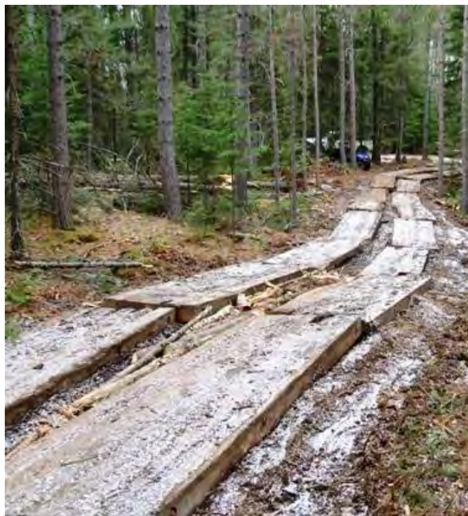
Figure 24 Planking utilized during spring thaw to prevent rutting and compaction
