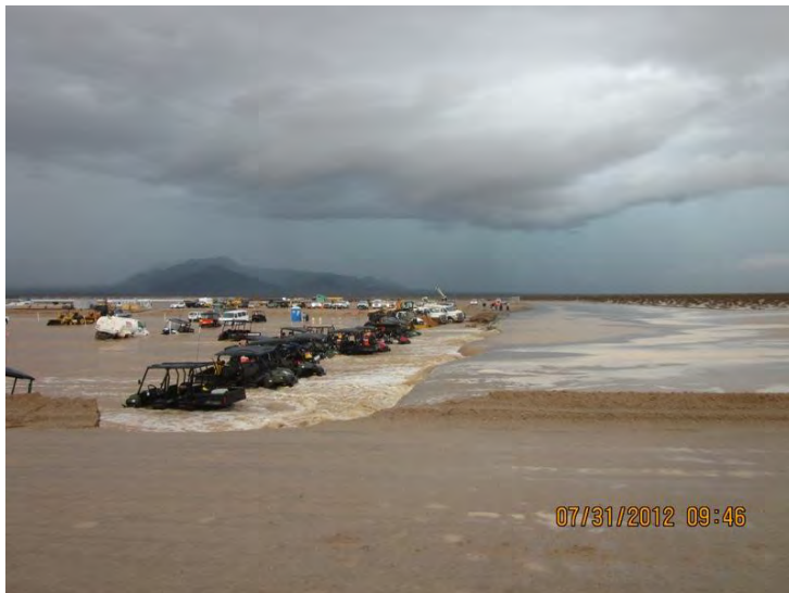
^The biggest flood took place at NextEra's Genesis Project on July 31 st , 2012. The close proximity to a dry lake and alluvial fans make this project location one of the poorest choices to site a large solar project.
