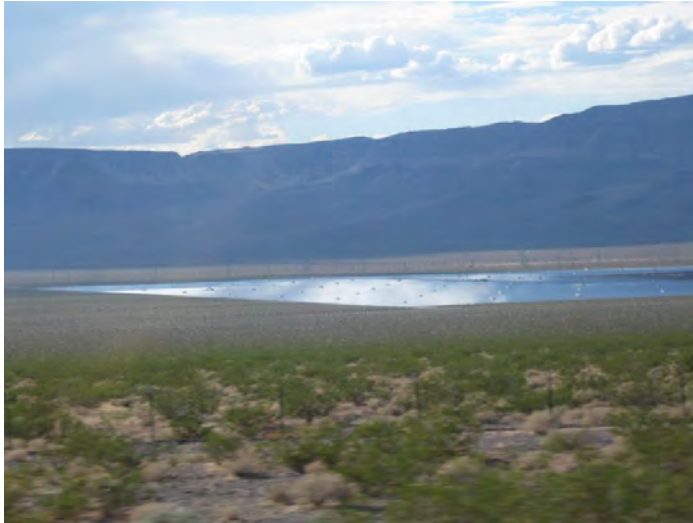
^Copper Mountain Thin Film Solar Farm, Boulder City, Nevada
