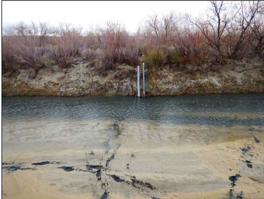
PHOTO 3.1. RIGHT BANK AT GAGING STATION G1 (A1 CROSS SECTION 9)
