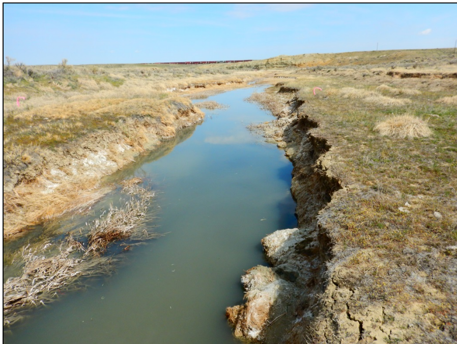
PHOTO 2.36. SITE A5 LOOKING DOWNSTREAM AT CROSS SECTION 5
