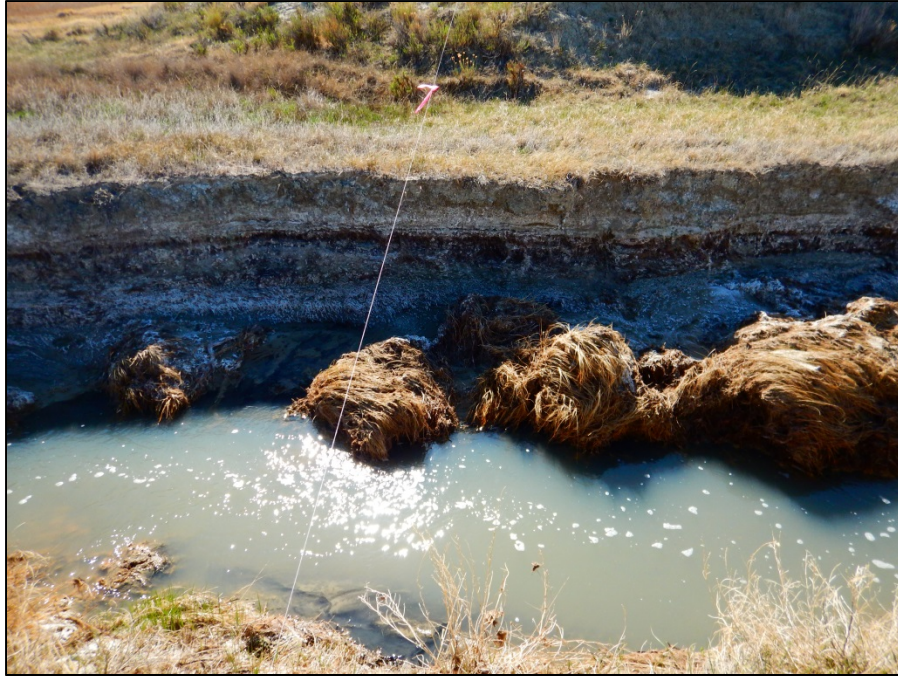
PHOTO 2.23. SITE A3 LOOKING AT LEFT BANK OF CROSS SECTION 3 NOTE SHEAR BLOCK FAILURE
