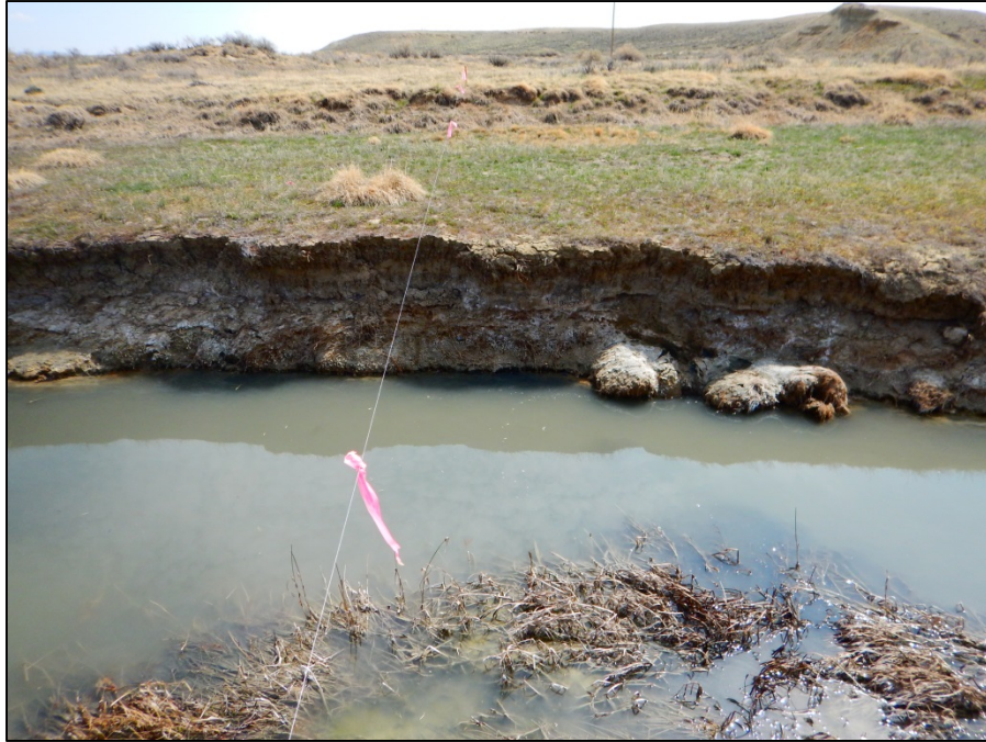
PHOTO 2.35. SITE A5 LOOKING AT RIGHT BANK OF CROSS SECTION 5
