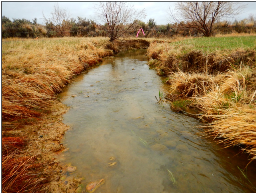
PHOTO 2.12. SITE C1 LOOKING DOWNSTREAM FROM CROSS SECTION 7 SHOWING MINOR BANK EROSION ON LEFT BANK NEAR CROSS SECTION 6
