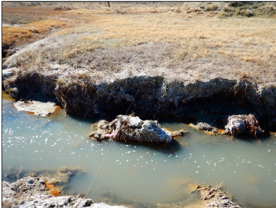
PHOTO 2.24. SITE A3 LOOKING AT LEFT BANK OF CROSS SECTION 4 NOTE SHEAR BLOCK FAILURE
