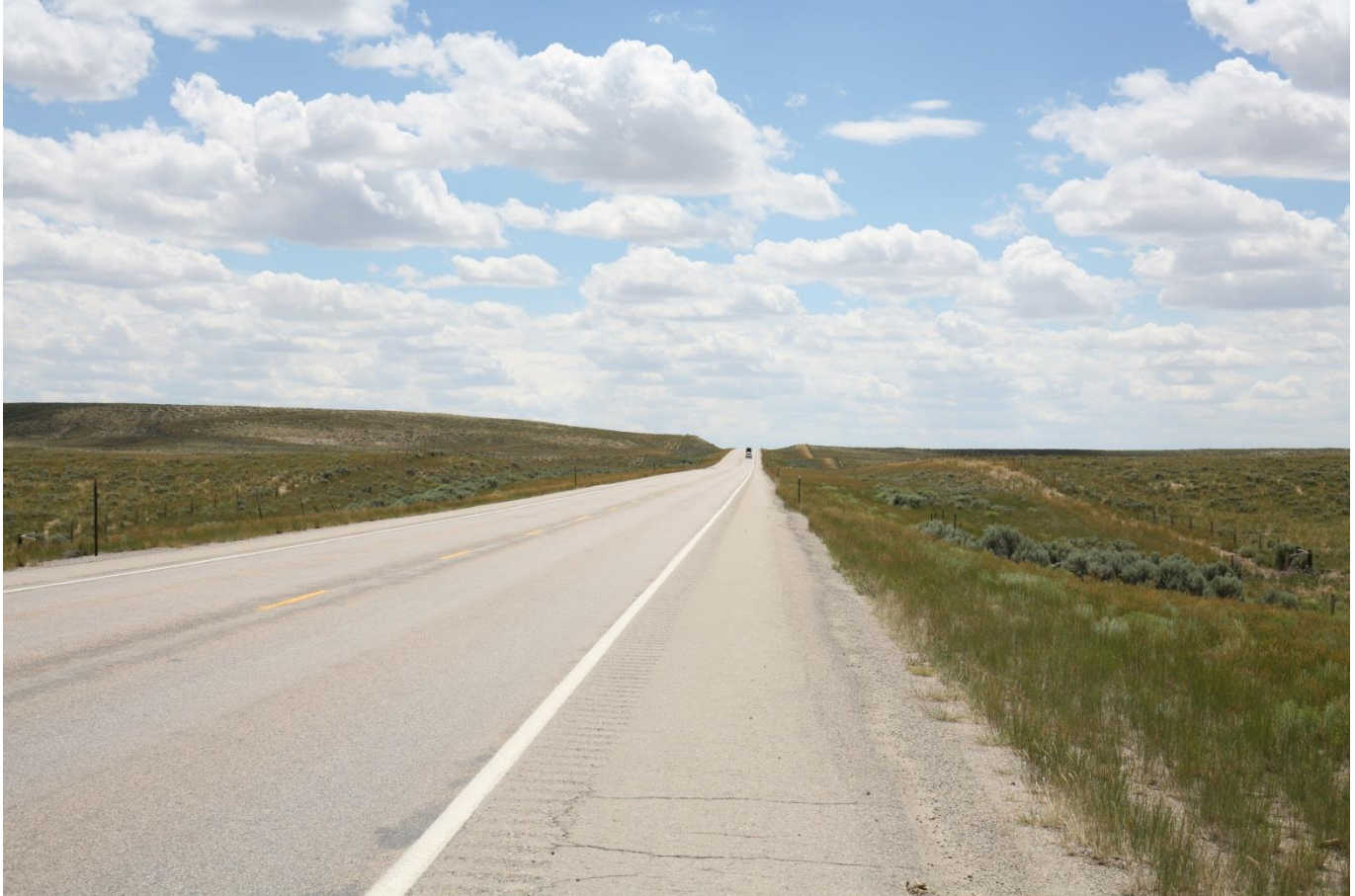
Photo taken toward the south on U.S. Highway 191 facing Southern Route Alternative
