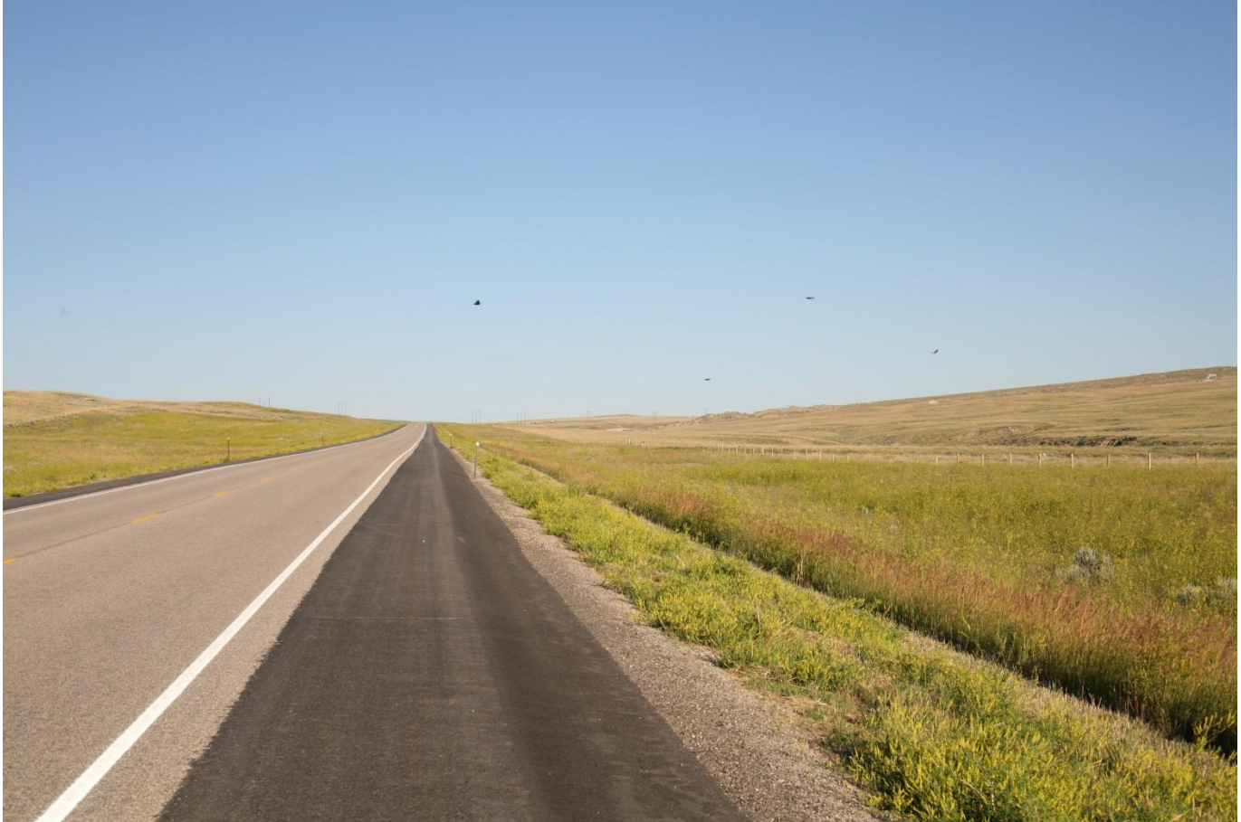
Photo taken facing west on U.S. Highway 20, Segment 3C parallel to road
