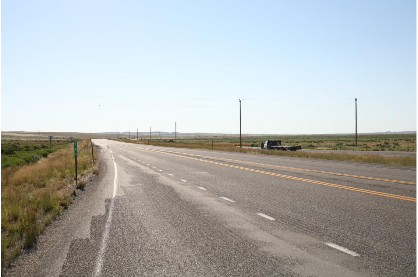
Photo taken facing east on U.S. Highway 20, Segment 3C parallel to road
