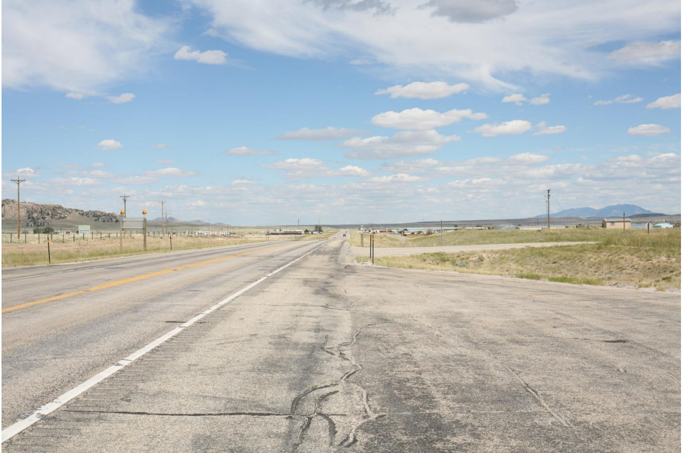
Photo taken toward the east on pull off on U.S. Highway 287 towards Segment 3B
