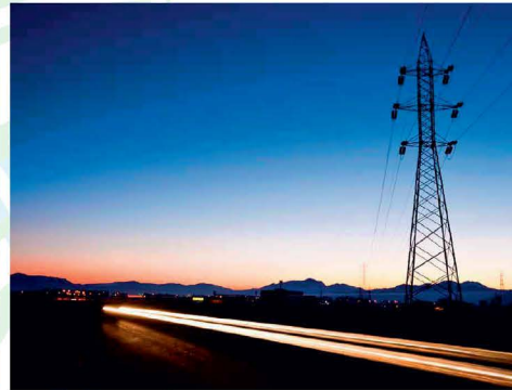
Transmission line adjacent to road
