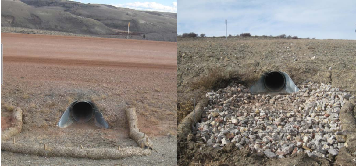
Figure 5. Example CMP Culvert Crossing
