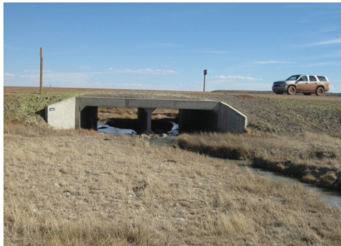
Figure 6. Example Concrete Box Culvert Crossing
