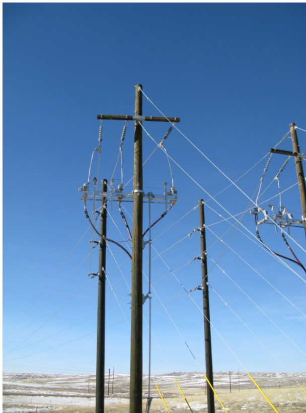
Figure 4-19. Example Riser Pole Structure
