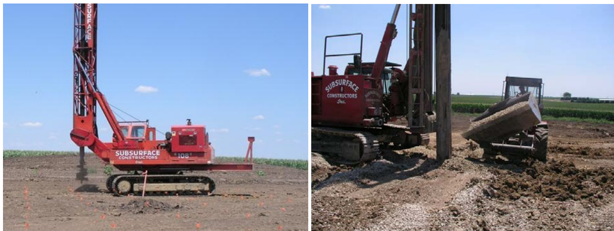
Figure 4-10. Stone Column Installation
