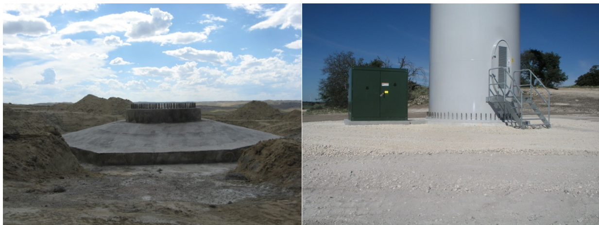
Figure 4-6. Wind Turbine Foundation Examples
