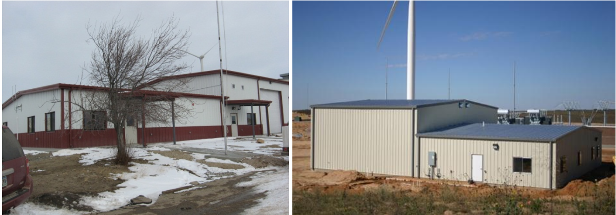
Figure 4-23. Example Wind Energy Maintenance Buildings
