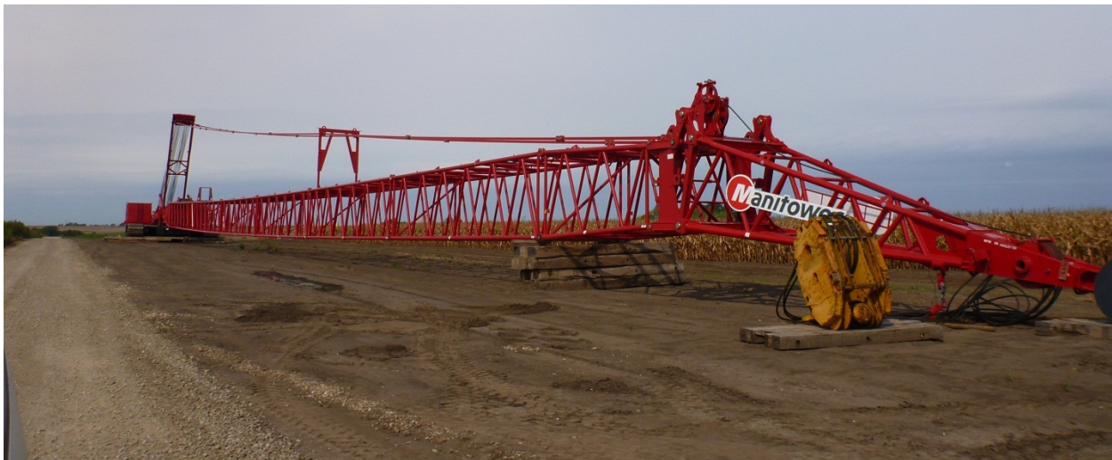
Figure 4-29. Crane Assembly Area
