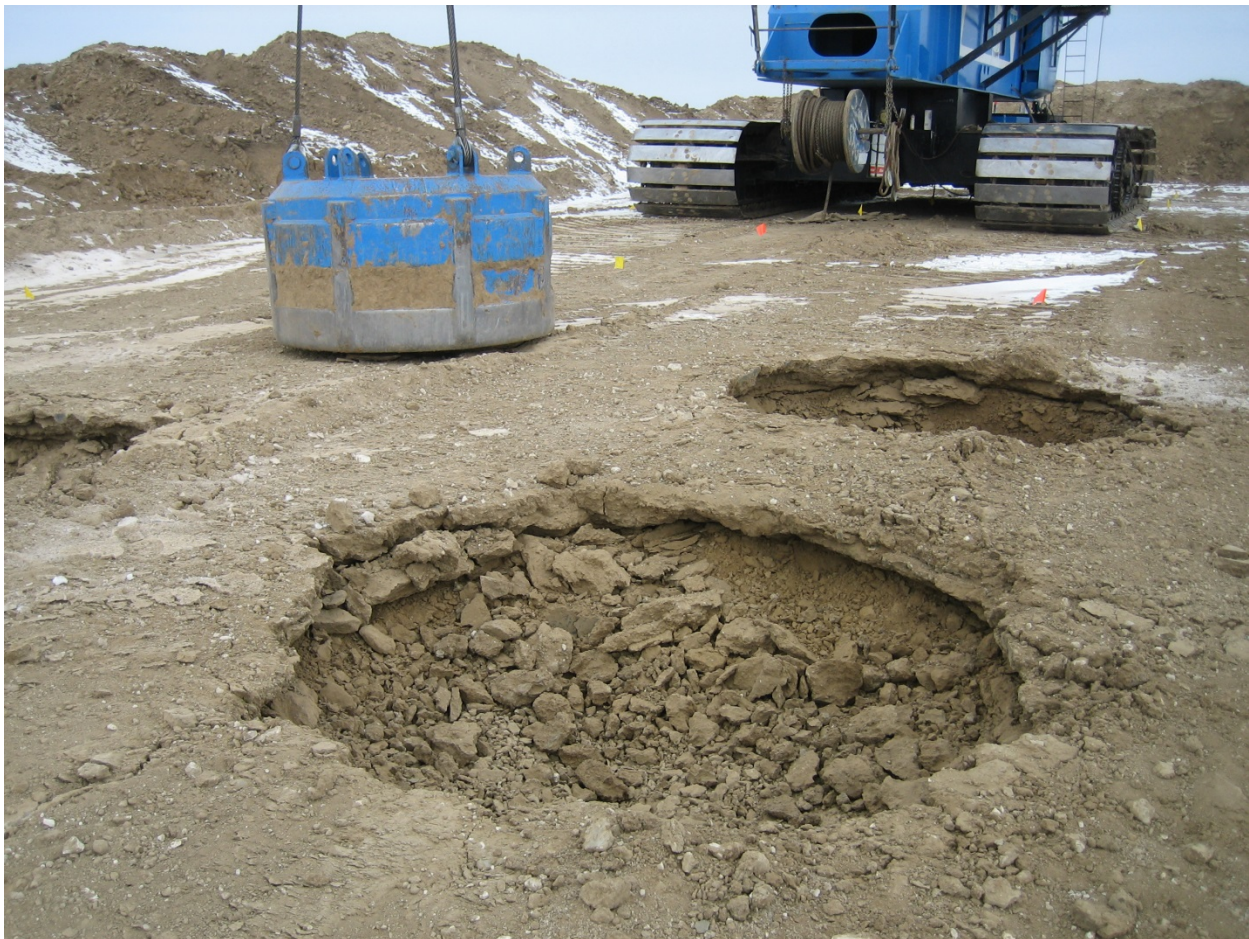
Figure 4-11. Dynamic Compaction
