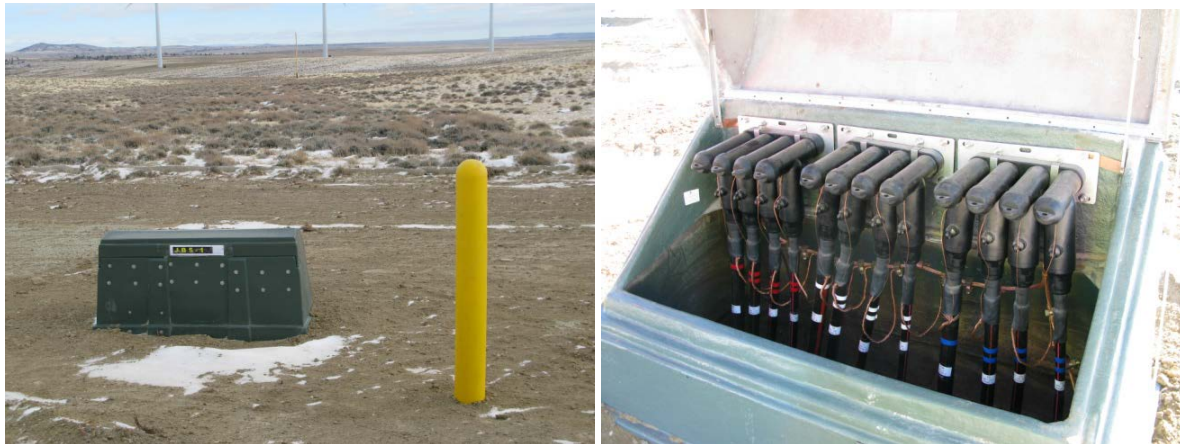
Figure 4-18. Examples of Junction Boxes
