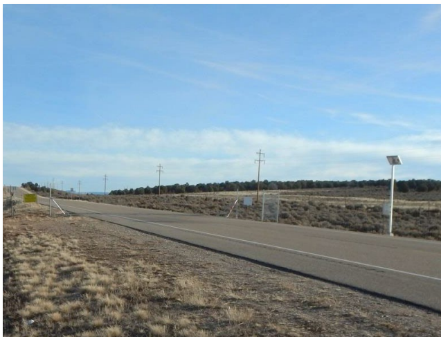
View Eastbound along U.S. Highway 89
