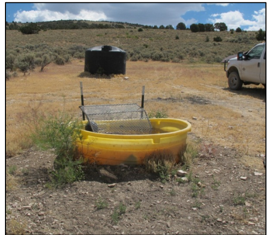
McCullough Springs water haul, July 2014. A 3000 gallon storage tank keeps the trough full with use of a float.
