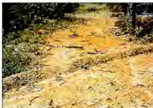
Figure 1—A water bar effectively intercepts the surface water and diverts it from the road
