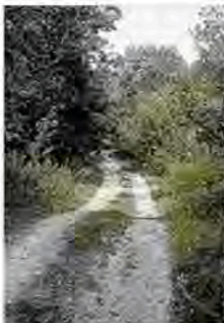
Figure 4—Broad-Based Drainage Dip
