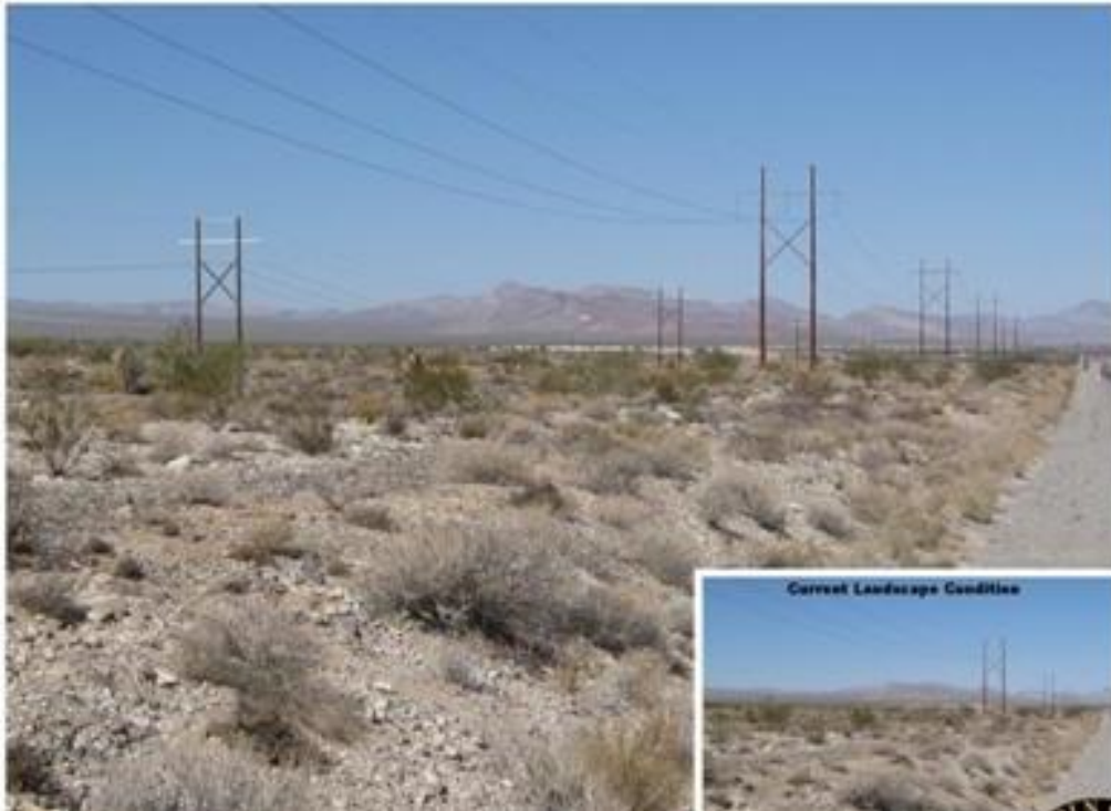
Figure 4.1 Photo-simulation of the visual effects of the new H-frame transmission structures paralleling the existing 69kV transmission line and highway US 93 in Coyote Spring Valley (photo by M. Cablk and J. Miller of DRI; photosimulation by ECI)
