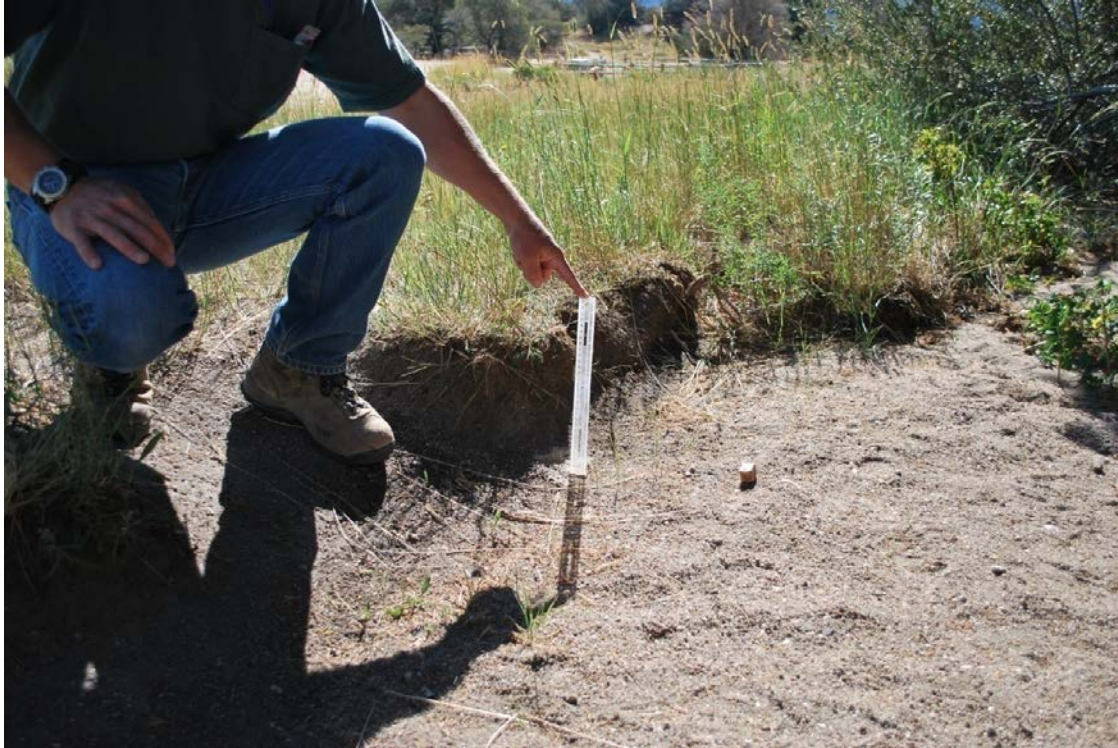
Figure 1. Loss of soil at staging area at City of Rocks Preserve (08/26/09).
