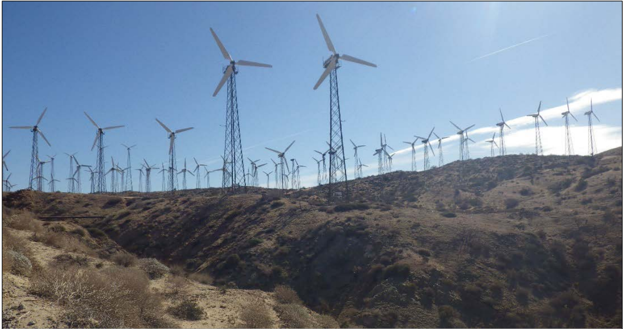
Figure 5. Vesta Turbines on Steel Lattice Trestles at the Mesa Wind Facility
