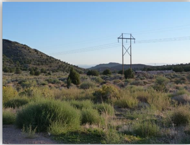
KOP 1 Figure: View to the south from KOP 1 at the existing conditions.
