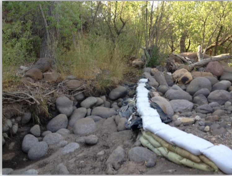
Figure 3-5: View to the north at the existing diversion on South Ash Creek, July 9, 2012. This sandbag diversion is rebuilt as needed by the Pintura irrigation users. The existing on-stream diversion berm beneath the sand bags is evidence of the long-term, historical diversion efforts.
