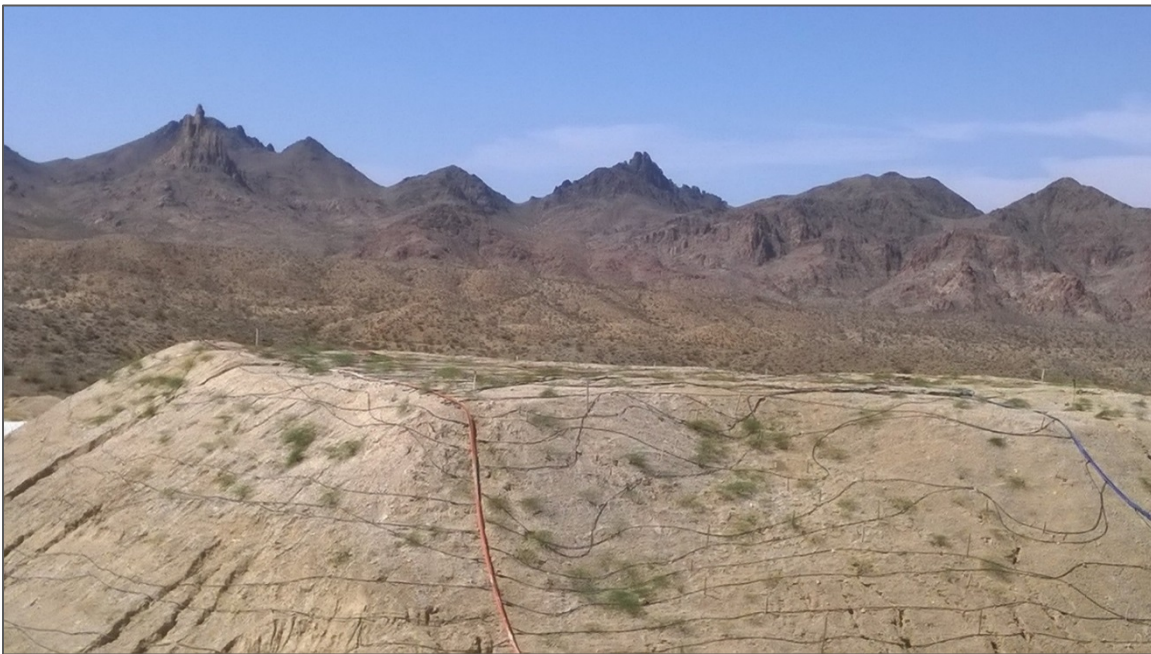
Photograph 3: Phase I Leach Heap Pad Revegetation
