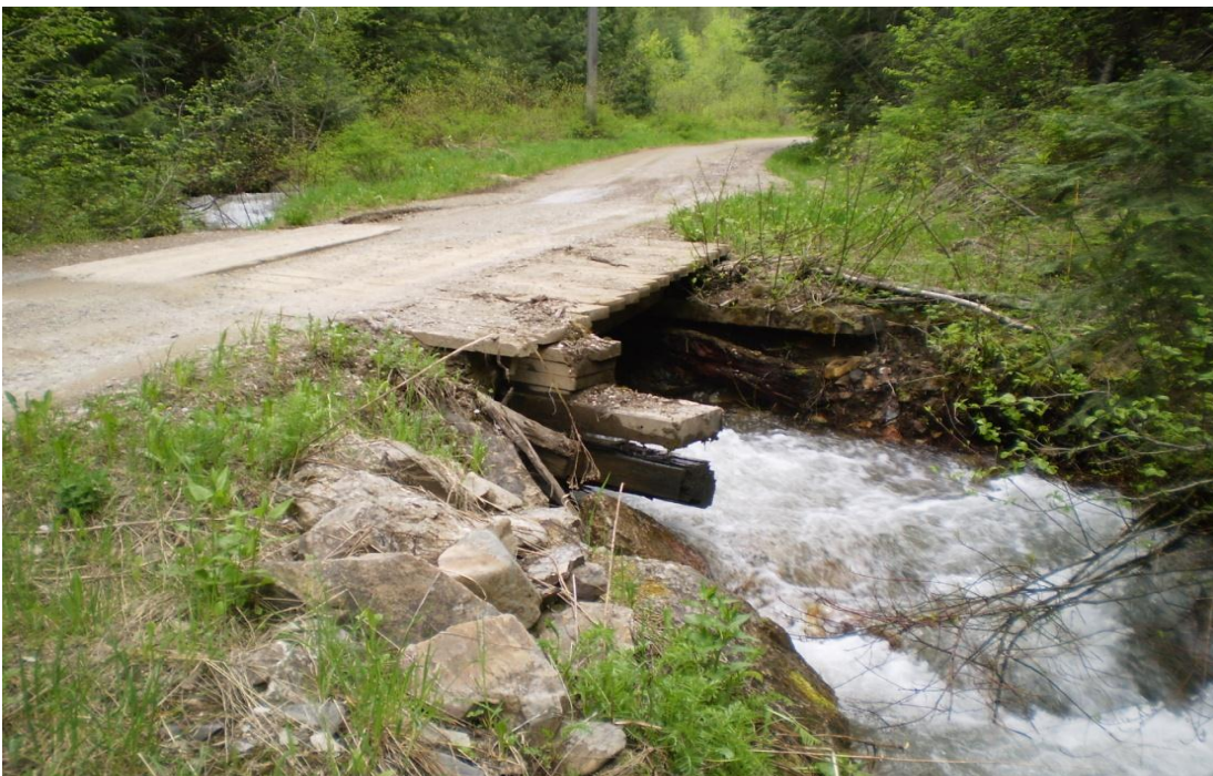
Photo 2. A picture showing the existing wooden bridge located on Mill Creek.
