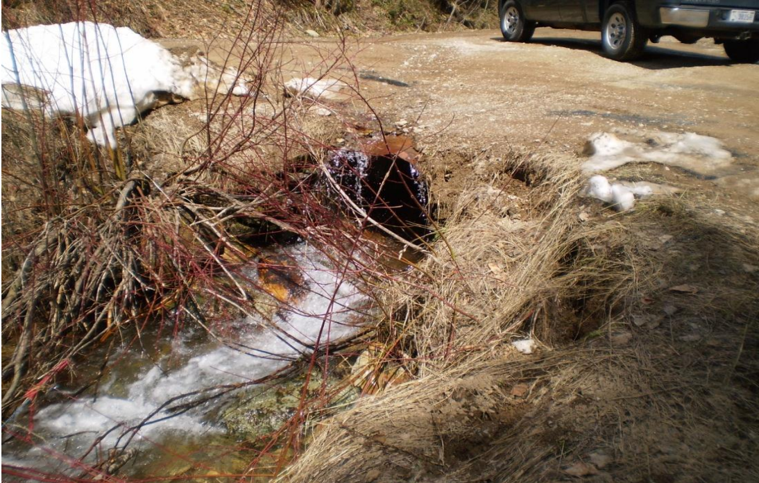
Photo 1. A picture showing the existing culvert located on Mill Creek.
