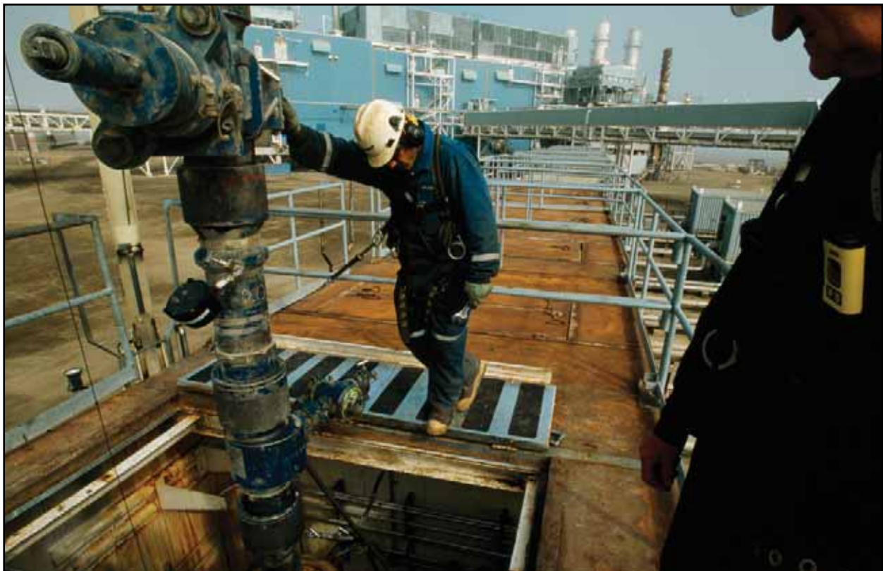
Oil workers perform a 'work over' on a thirty-year-old well head in Prudoe Bay.
