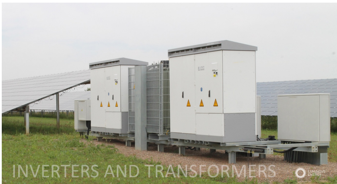
FIGURE 1-5 PHOTOGRAPHS OF A TYPICAL POWER CONVERSION STATION/INVERTER
