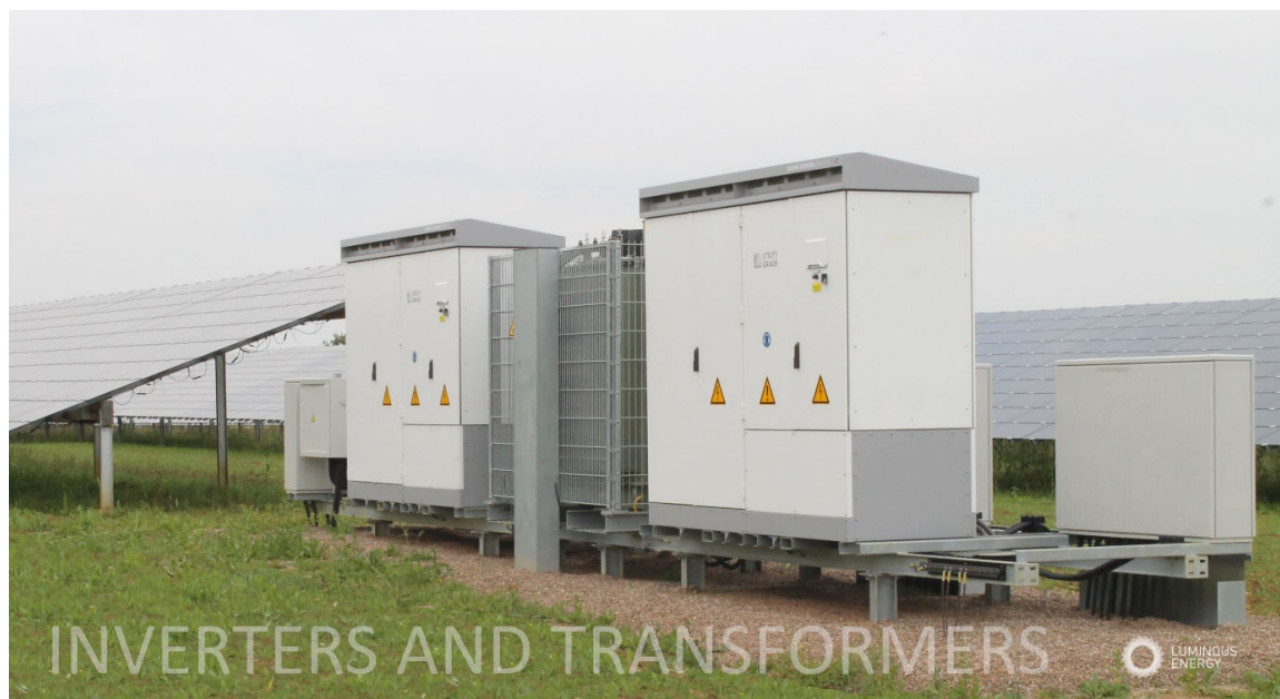
FIGURE 1-5 PHOTOGRAPHS OF A TYPICAL POWER CONVERSION STATION/INVERTER
