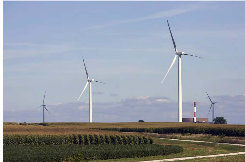
Grand Ridge Wind Energy Center. GE 1.5-MW turbines in Lasalle County, Illinois. Photo by Invenergy, LLC, NREL 16040.
