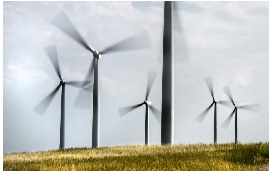
Combination of 221 Mitsubishi Heavy Industries 1-MW turbines and 53 GE 1.5-MW turbines at the Cedar Creek Wind Farm in Grover, Colorado. Photo by Dennis Schroeder, NREL 30593
