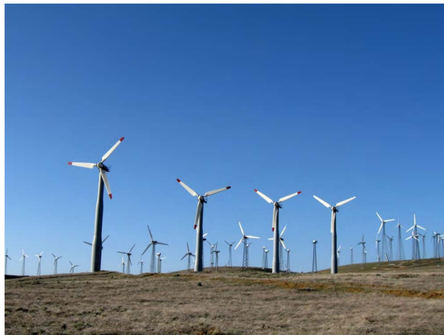
705-MW project in Tehachapi Pass Wind Resource Area, California.
