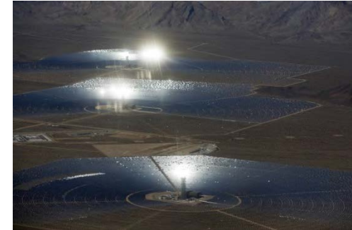
Ivanpah Solar Electric Generating System
