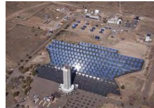
National Solar Thermal Test Facility (NSTTF)
