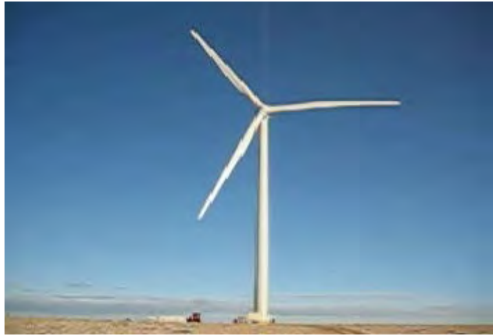
93-m diameter RSA and 2.5 MW
