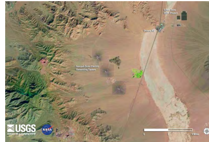
Ivanpah Solar Electric Generating System
