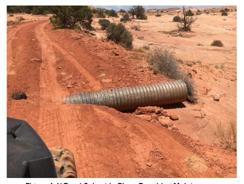
Figure 4. V-Road Culvert in Place Requiring Maintenance
