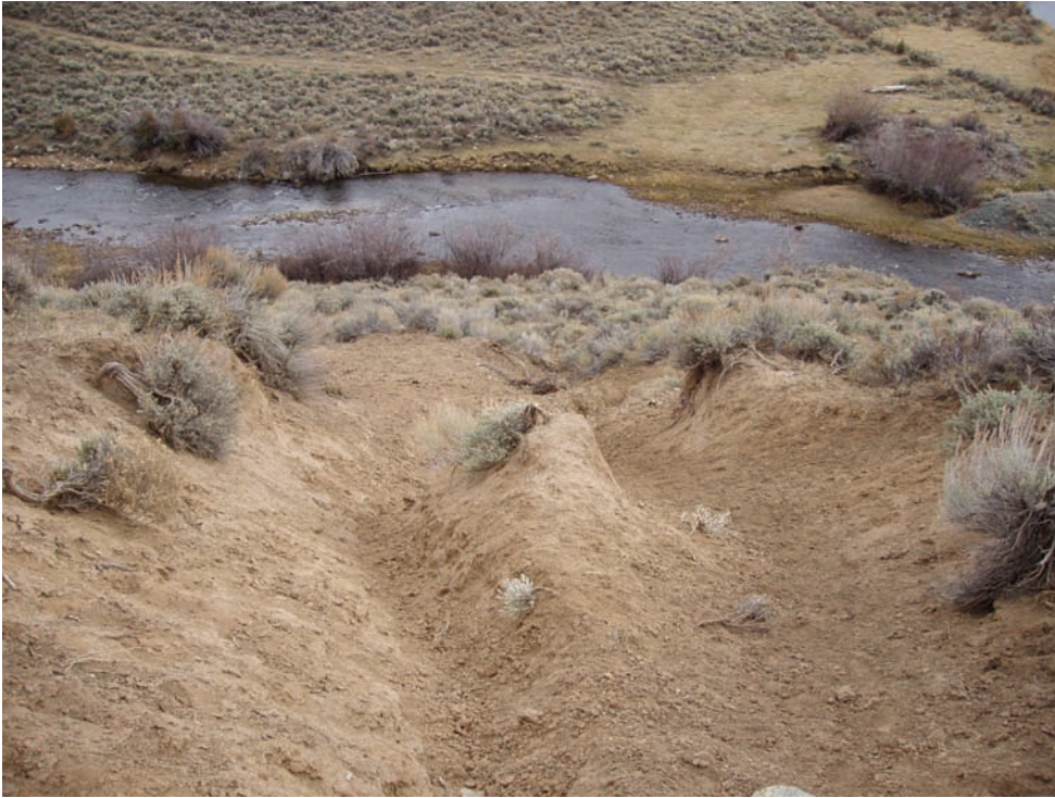
Page 29-2 Gully erosion into Big Creek, Platt Mine Allotment
