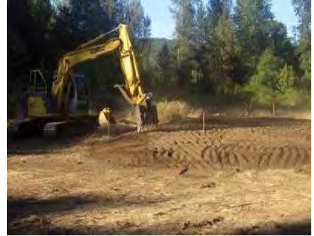
Figure 3-18: An Excavator Moves Nesting Material into Place
