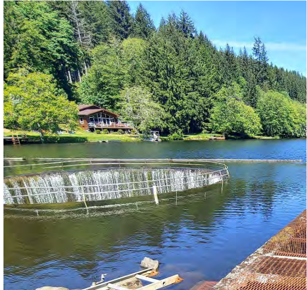
Figure 2-2. A Morning Glory Spillway at Fishhawk Lake
