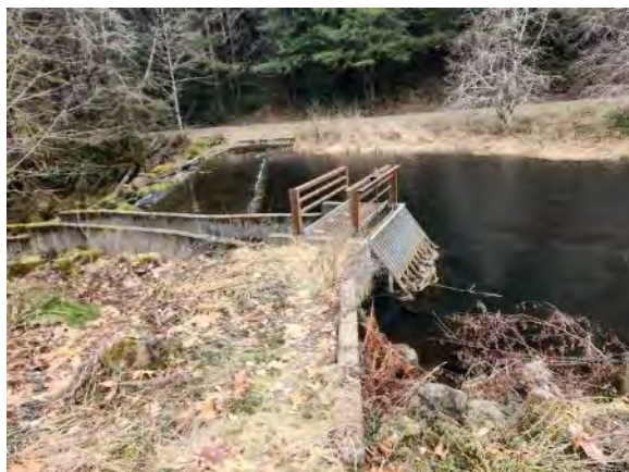
Fish ladder trash rack and spillway crest from spillway dike. Outlet conduit with leakage.
