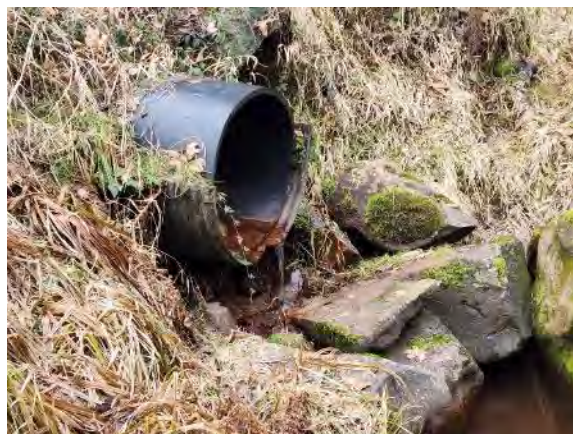
Fish ladder trash rack and spillway crest from spillway dike. Outlet conduit with leakage.
