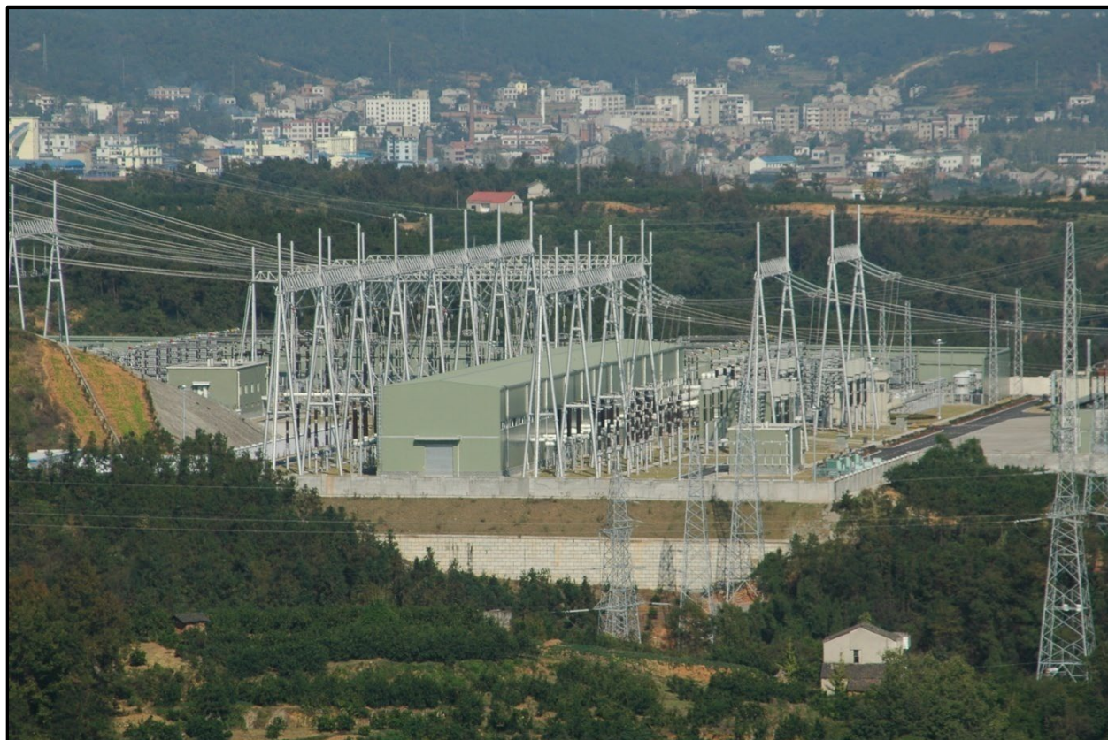
FIGURE 11A TYPICAL AC/DC CONVERTER STATION
