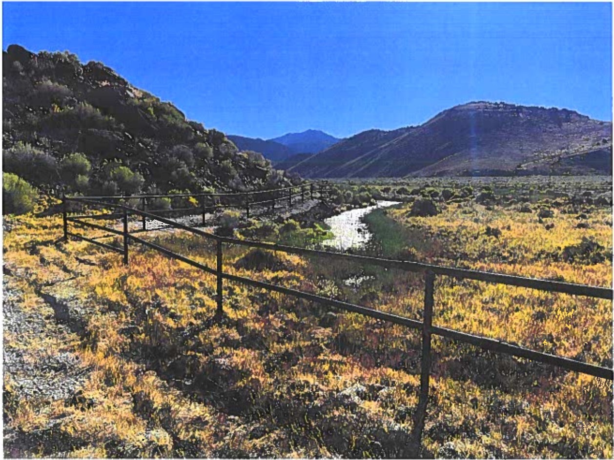
Figure 4. An example of the welded drill steel exclusionary fencing.
