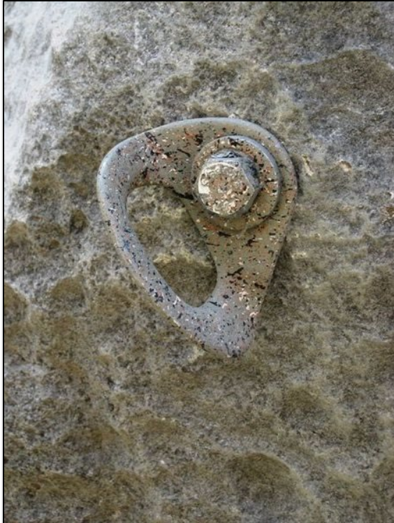
Figure 1. Example of camouflaged bolt and hanger. P.C. mountainproject.com
