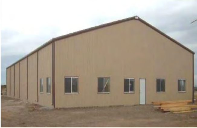
Figure 1-8. Typical Operations and Maintenance Building
