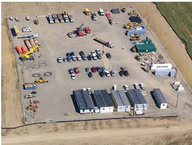
Figure 1-11. Typical Construction Laydown Area for Storage, Staging, Laydown
