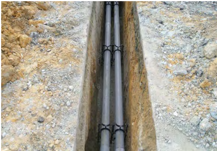
Figure 1-5. Typical Buried Collection Lines
