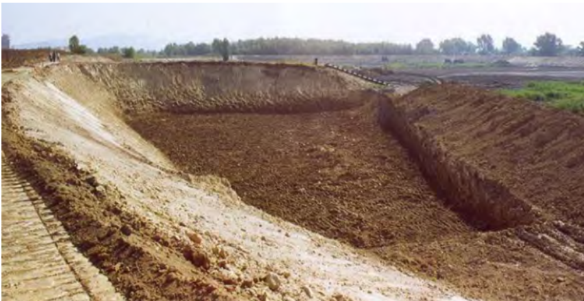
Figure 1-10. Typical Borrow Pit
