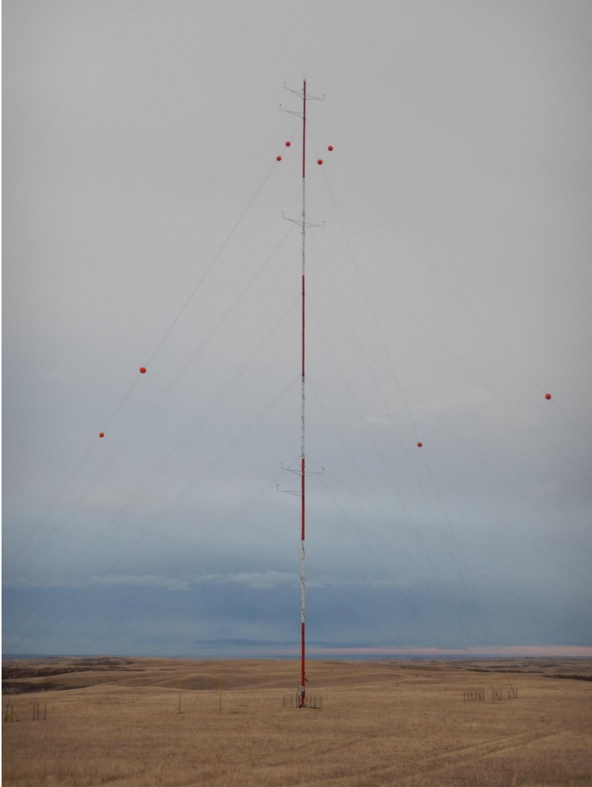
Figure 6 Typical 60M MET Tower with Marker Balls
