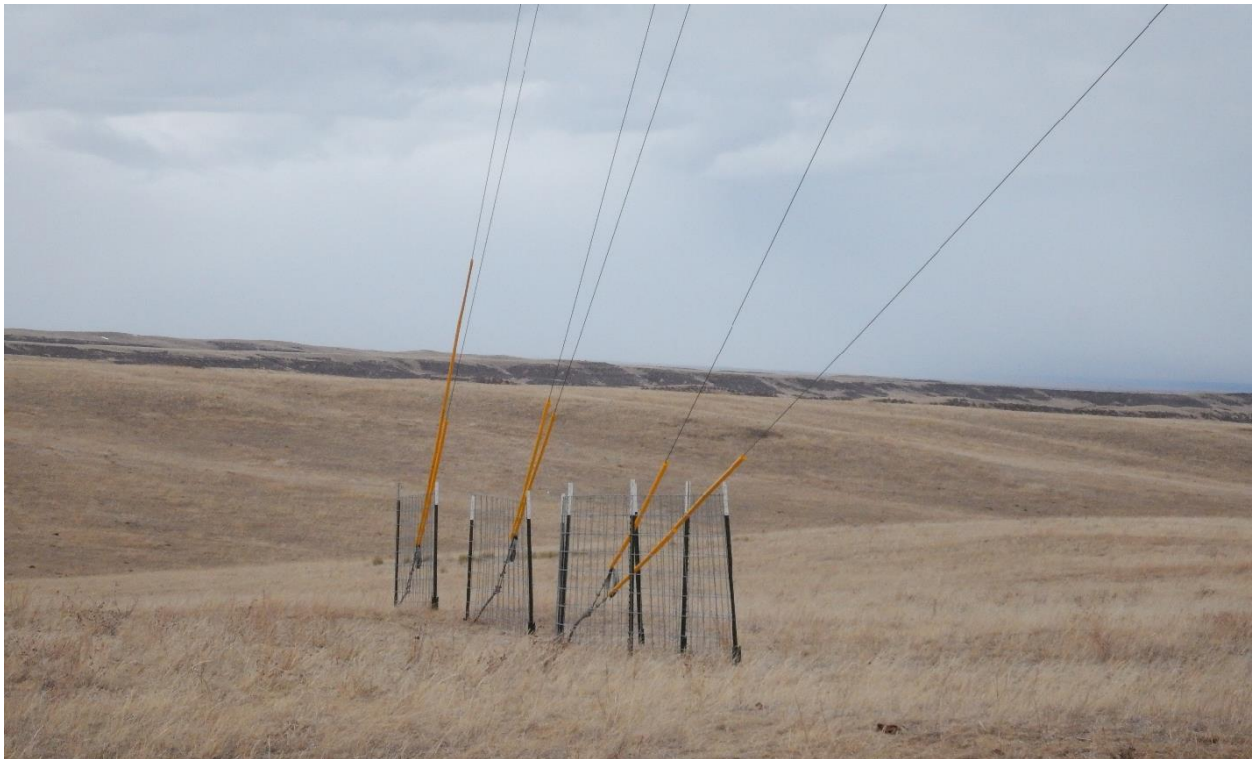
Figure 8 Typical 60M MET Tower Guy Wire Ground Anchors
