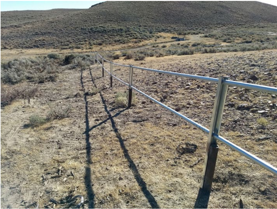
An example of a Steel Posts Driven into the Ground and Pipe style fence.
