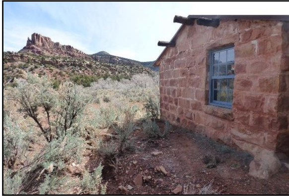
Figure J-2. North Cottonwood Guard Station.
