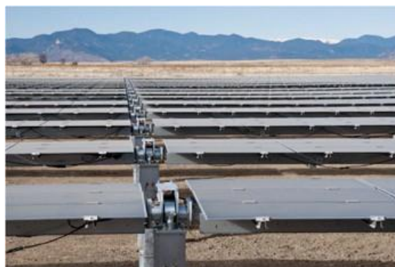
Typical Tracker Array Configuration and Mounting Systems
