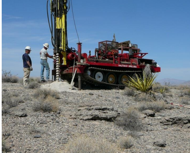
Figure 8. Typical Track-Mounted Drill Vehicle
