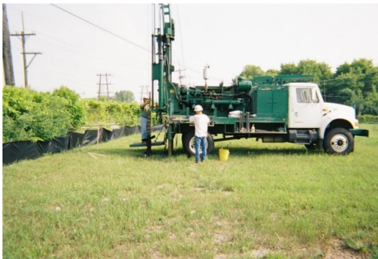
Figure 6. Typical Truck-Mounted Drill Vehicle
