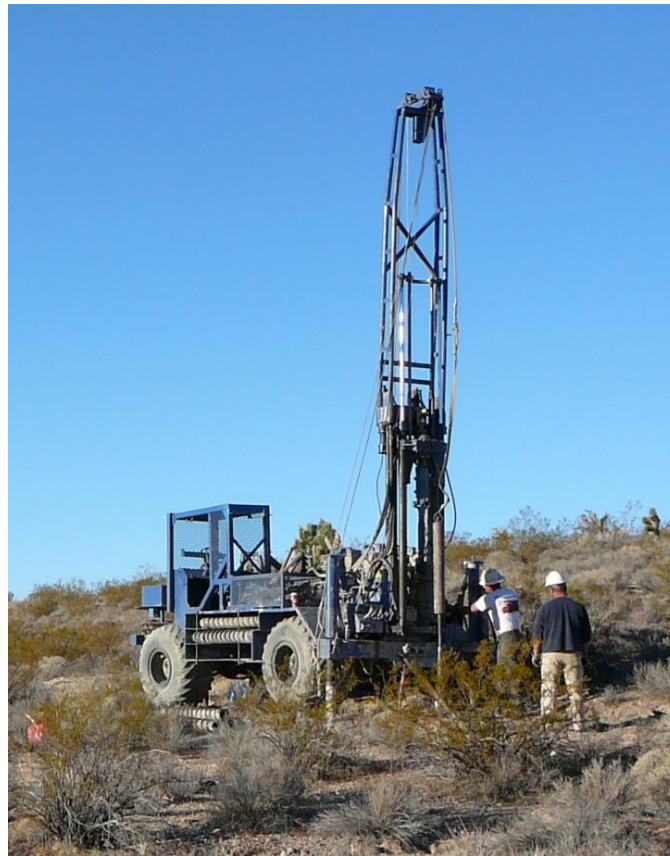
Figure 7. Typical ATV-Mounted Drill Vehicle
