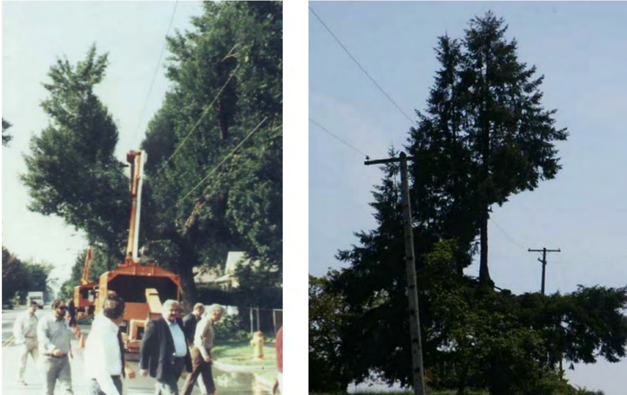
Figure 3.3 "V" or "L" shapes can develop from crown reductions on trees growing in close proximity to power lines. The ultimate objective is to train the tree up and away from the conductor whenever possible, so the facility is cleared while minimizing health risks to the tree.
