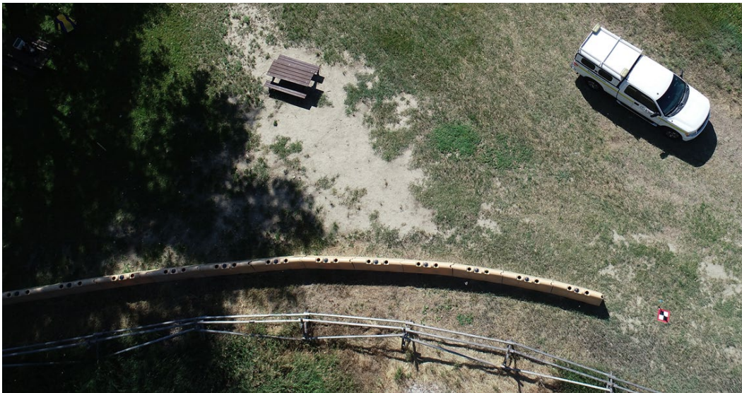
Figure 1 Southeast end of the barrier, prior to being extended.
