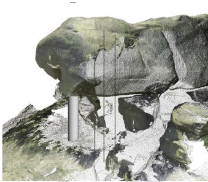
Figure 28 Rendering of the of the proposed underpinning stabilizing the Turtle Rock head.
