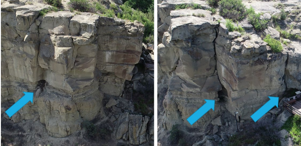
Figure 10 Siltstone weathering and erosion areas.
