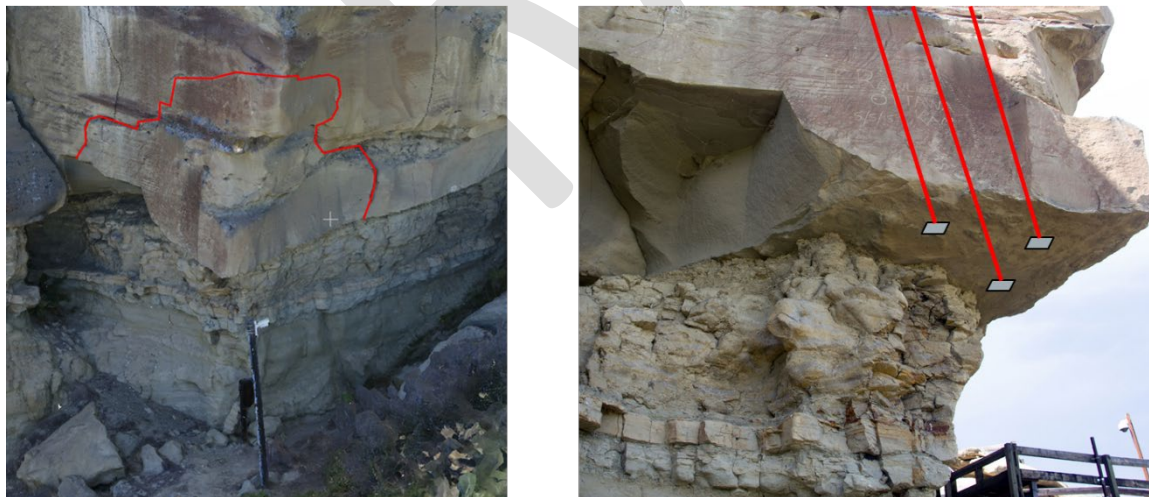
Figure 25 Signature Block 2a, 2b, and 2c rock bolting.
