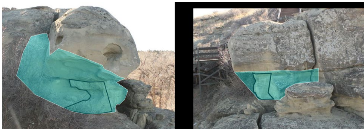
Figure 30 Full area of analysis of possible underpinning at Turtle Rock head.
