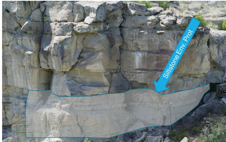
Figure 20 Extent of environmental protection of the siltstone.
