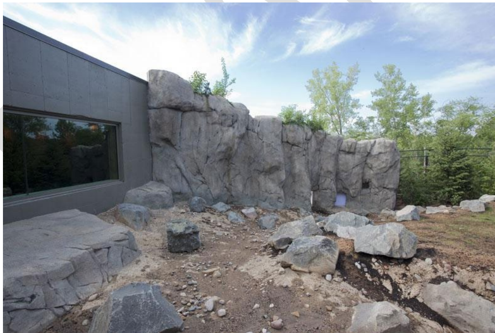
Figure 18 Example of concrete sculpting and coloring (left real rock, right concrete that has been colored to match then intentionally smoothed).
