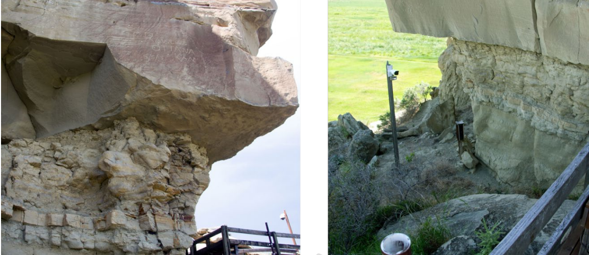
Figure 21 Two views of the Signature Block 2 overhang.
