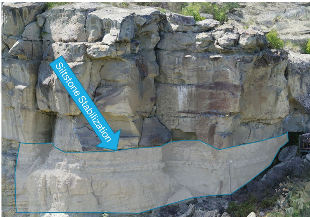
Figure 14 Approximate location and extent of siltstone stabilization.
