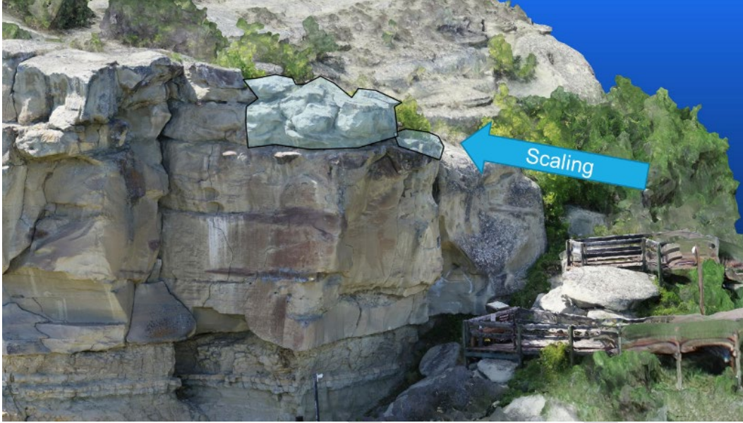
Figure 3 Likely scaling locations at the Signature Blocks area.
