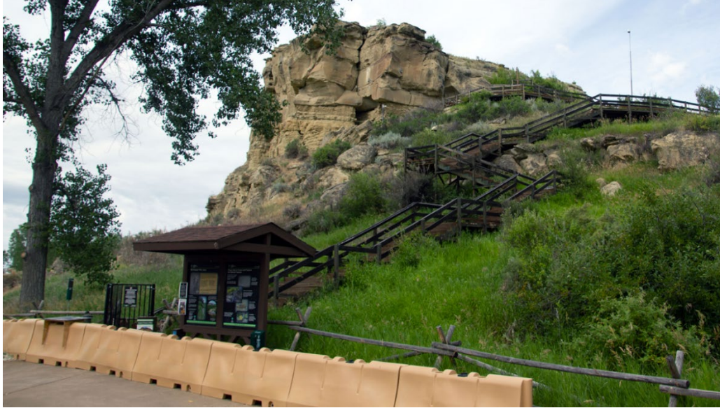
Figure 2 Northwest end of the barrier.
