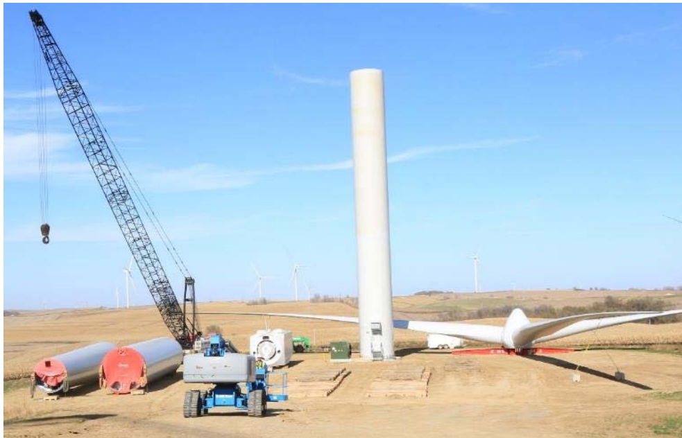
Figure 2-7: Erected Base Tower Section
