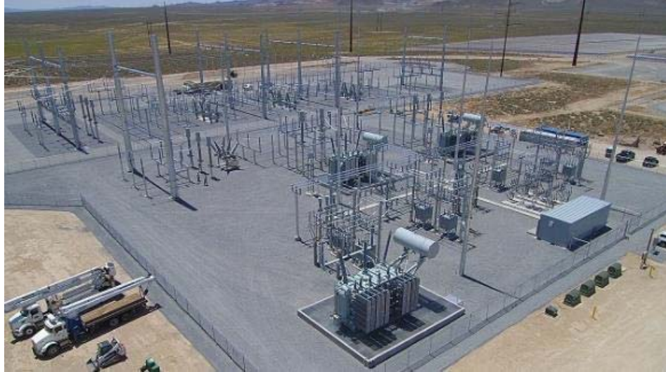
Figure 1-5: Example Collector Substation
