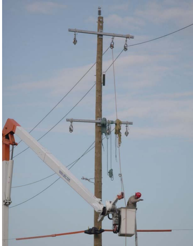
Figure 1-3: Typical Collector Line Structure
