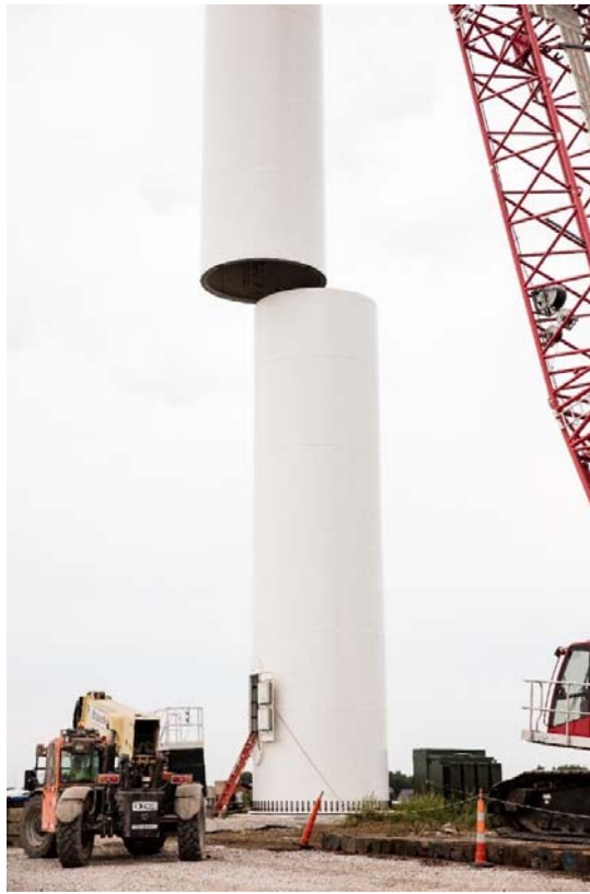
Figure 2-8: Mid Tower Section Placement
