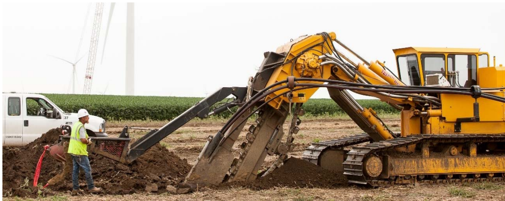
Figure 2-11: Typical Trenching with Trenching Machine
