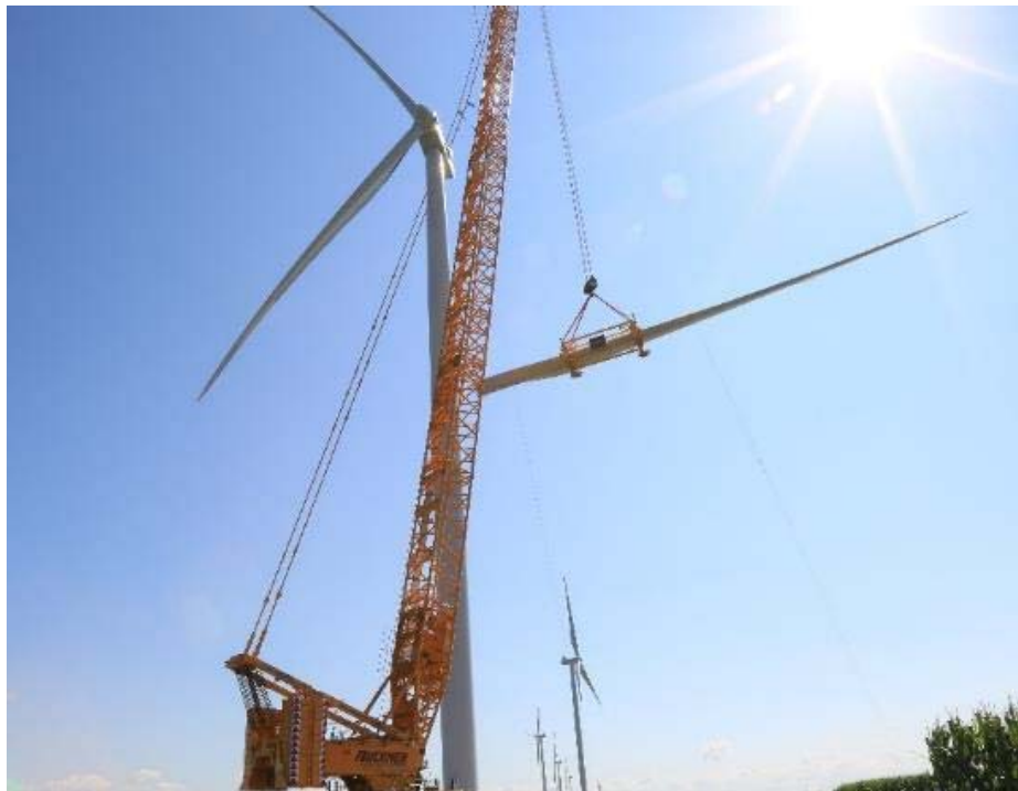
16 17 Figure 2-10: Crane Lifting Blade to the Hub
