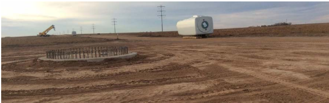
Figure 2-4: Backfilled Turbine Mat
