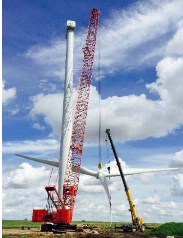
Figure 2-9: Erection of Complete Rotor
