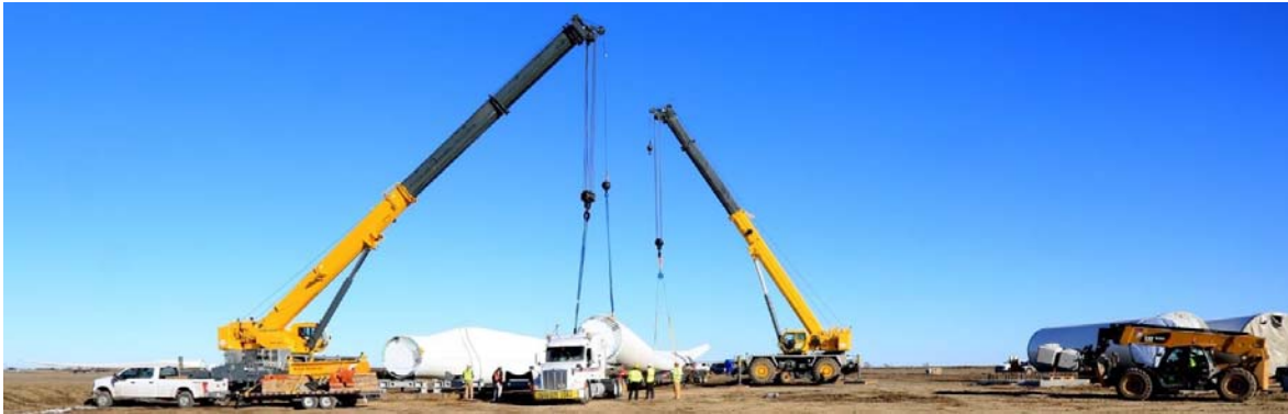
9 10 Figure 2-5: Typical Unloading of Turbine Components
