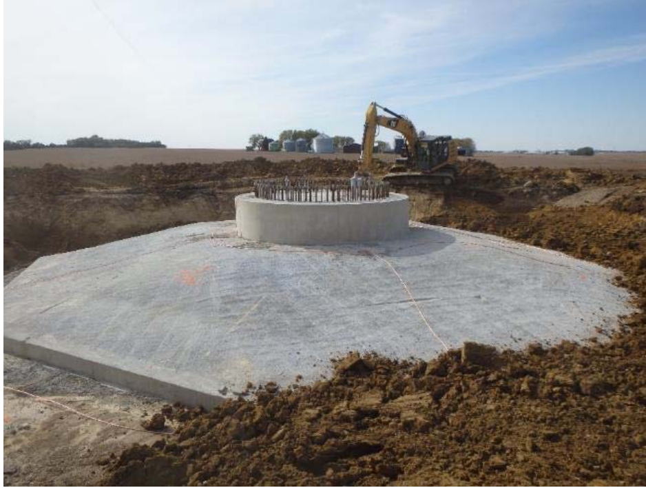
Figure 2-3: Complete Turbine Mat
