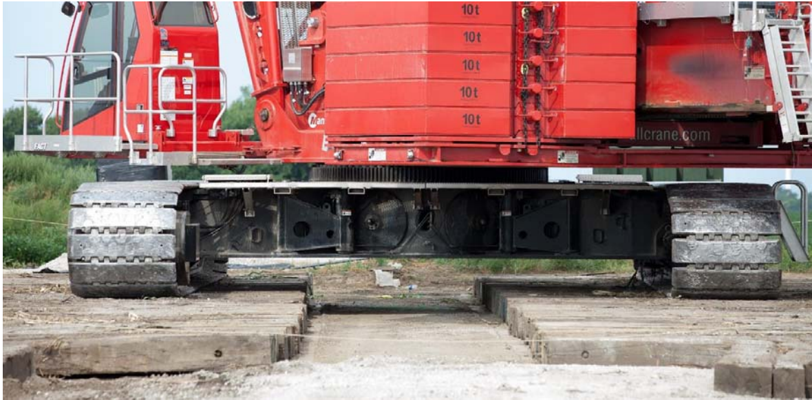
Figure 2-6: Crane Pad and Mats
