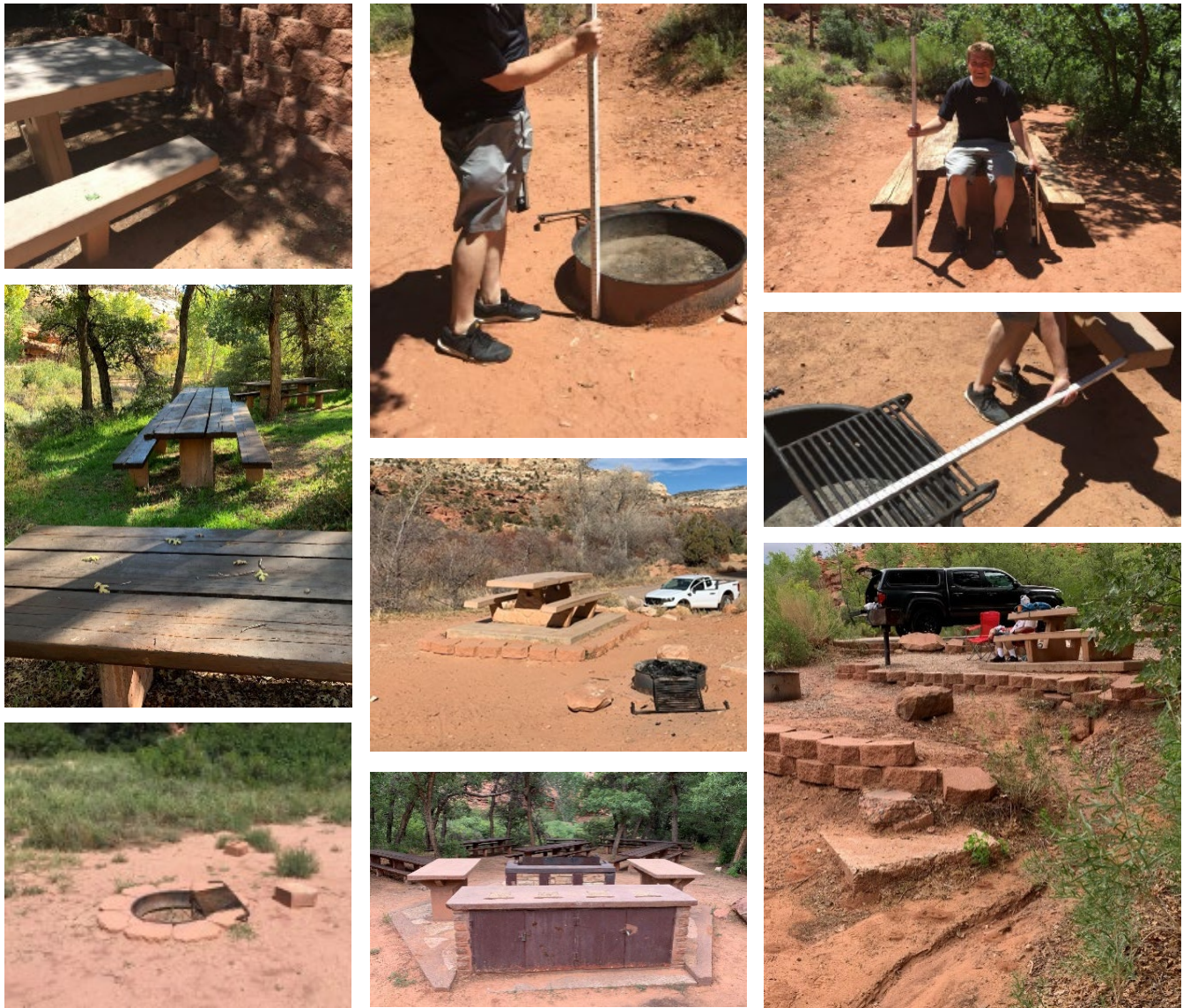
Figure 3 - Universal accessibility deficiency examples (top down, left to right): table too close to wall; group picnic tables that do not provide 19" of knee clearance; fire rings that do not provide 9" high fire building surface; table that is accessible on ends but that cannot be approached because of elevated pad surrounded by blocks; 1960s era grills and side tables that do not have required clear space; table that does not have 19" of knee clearance; fire ring and table that are too close together; campsite that is not universally accessible due to grade changes and erosion.
