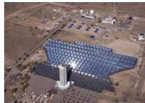
National Solar Thermal Test Facility (NSTTF)
