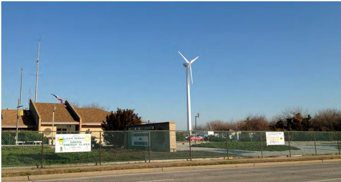
Northwind 100, 100-kW wind turbine; Hempstead, New York. Photo by Town of Hempstead, NREL 28963
