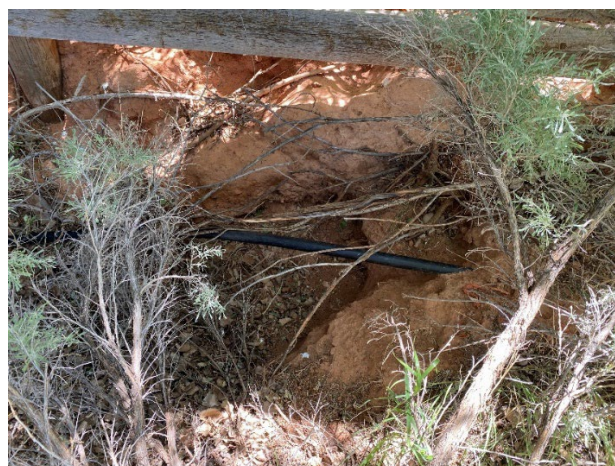
Figure 15: Incised channel forming near enclosure fence at Sykes Spring is exposing pipe infrastructure that was installed to convey water down spring.
