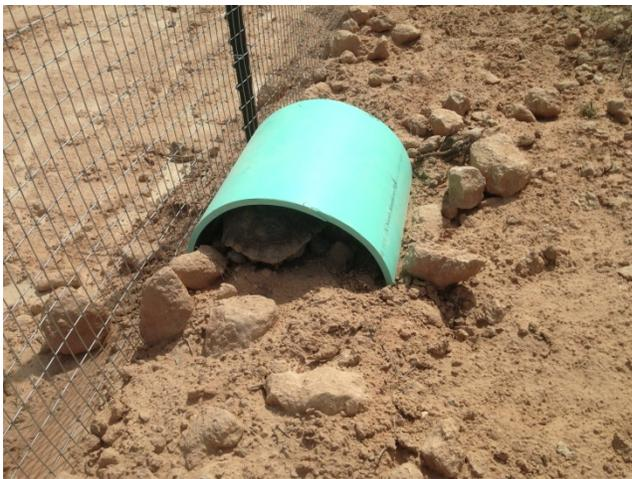
Photo 3: Schedule 80 PVC pipe, approximately 18 inches in length, no soil/rocks on top of structure. This is an example of a structure that is poorly constructed and could potentially be lethal to desert tortoises. Without adequate soil/rock insulation on top, radiative heat could be detrimental to desert tortoises inside the structure. The structure may also be too short to provide adequate cover for multiple animals or individual animals throughout a day.
