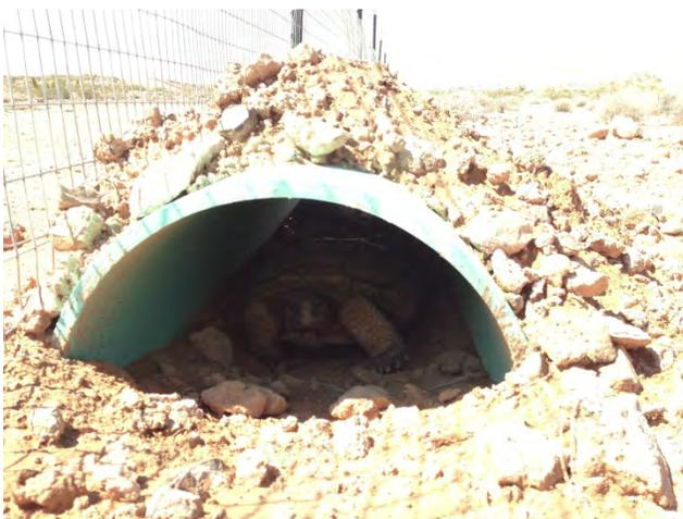
Photo 1: Schedule 80 PVC pipe, 6-feet in length, 3-4 inches of soil/rocks on top to insulate the structure. This is an example of an effective and durable structure.
