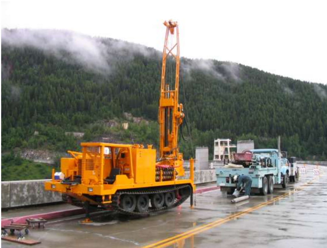
Figure 4 – The CME-850X track carrier mount with drill rig attached.
