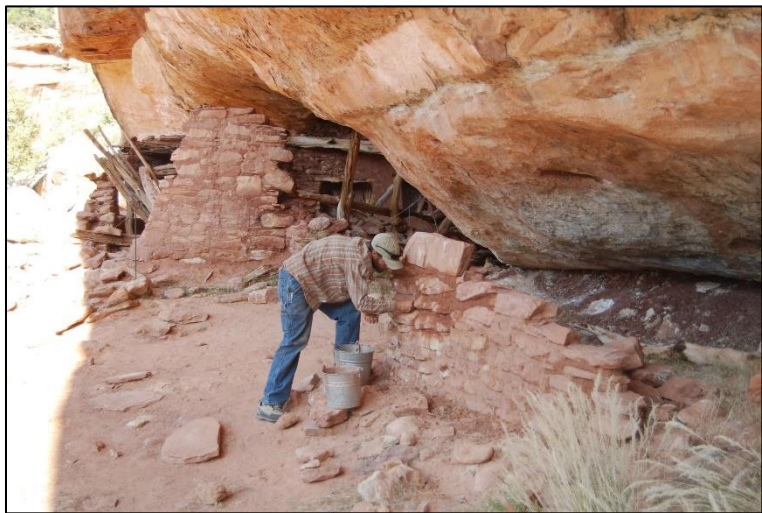
Stabilization project at Moon House
